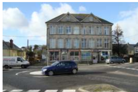
Figure 1.6 - Roche's historic square has been reduced to a roundabout
